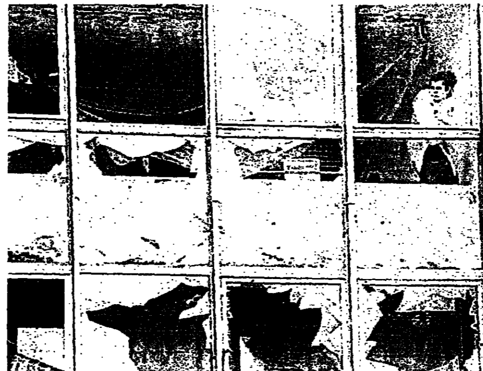
A Bosnian woman gazes from the shattered windows of a block of flats. Damaged but repairable homes are being destroyed to prevent refugees returning to them.
